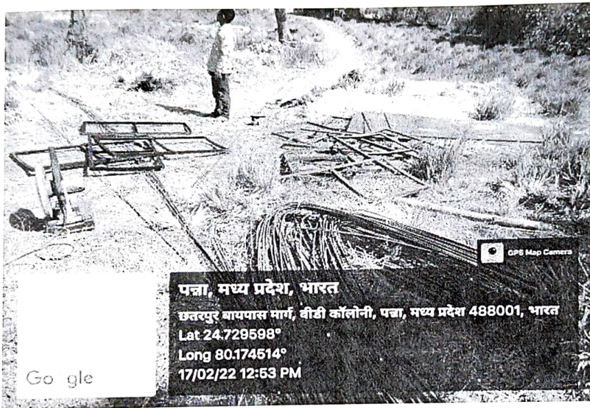
Fig. 2.5 Available reinforcements on site
