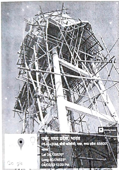
Fig. 1.2 Water tank construction
