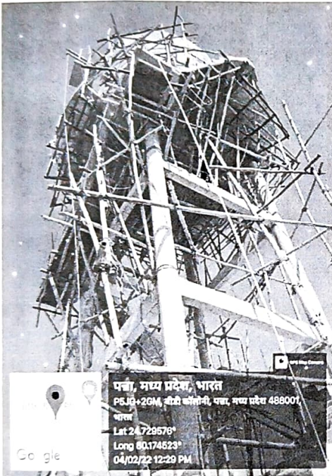
Fig. 1.2 Water tank construction
