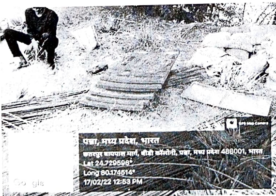
Fig. 2.4(A) Shuttering material on the site
